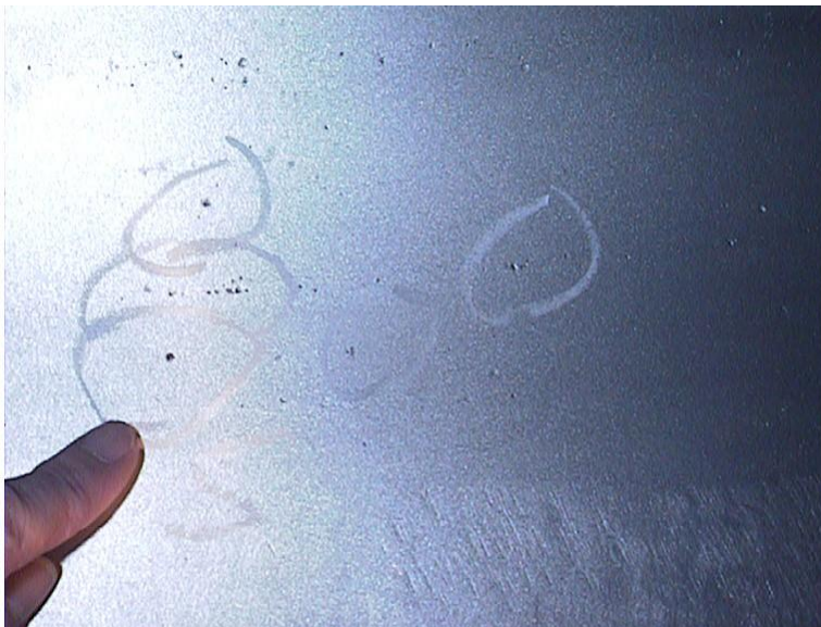
Figure 23: Cleaning level 3.6.x.x Pitting in the wall
