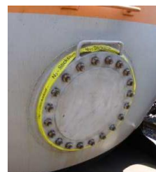
Example 6: screwed manhole gas
